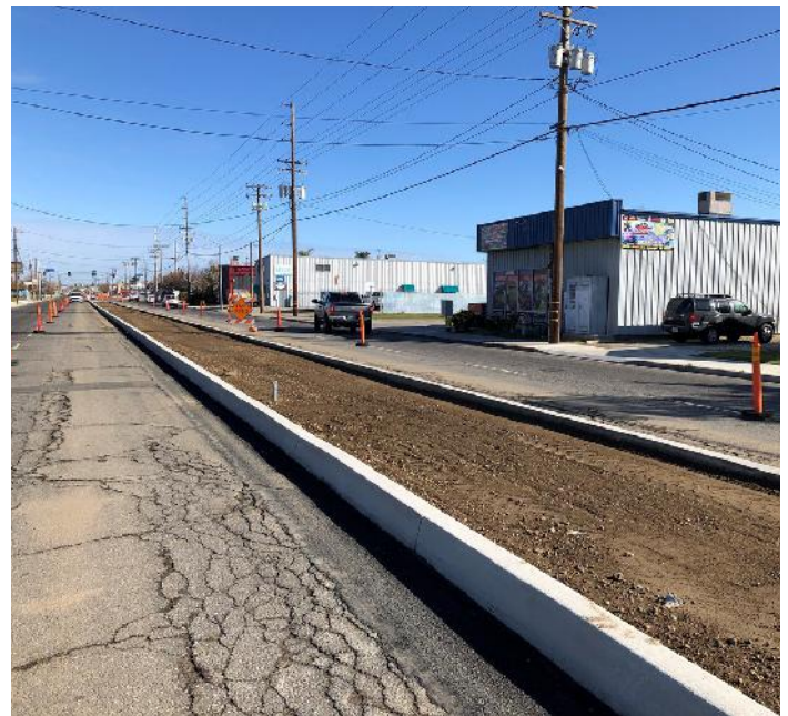
Photos from of median installation on City Project 21-018
